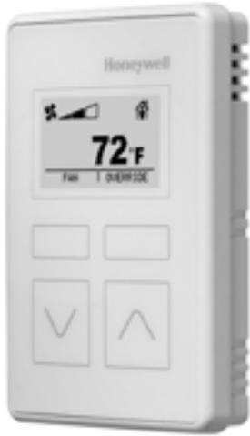
The TR40 and TR42 are 2-wire, non-polarity sensitive, Sylk bus communicating wall modules, which communicate with Spyder® and some ComfortPoint™ programmable controllers.
